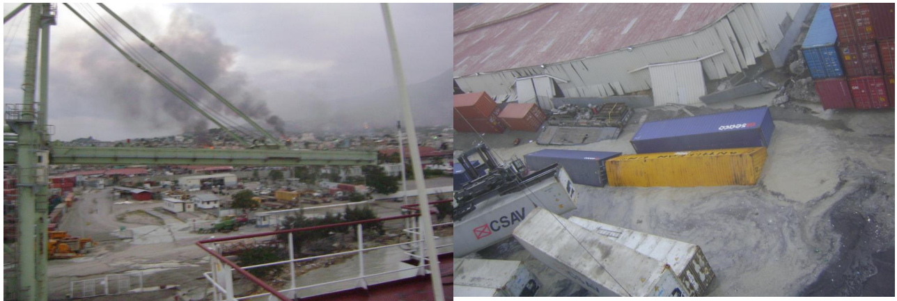
Photos of Haiti's damaged infrastructure in the days immediately following the earthquake.
